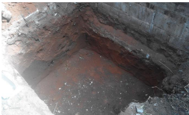
From left leach pit hole before and after the insertion of blocks, CFHD, 2022
