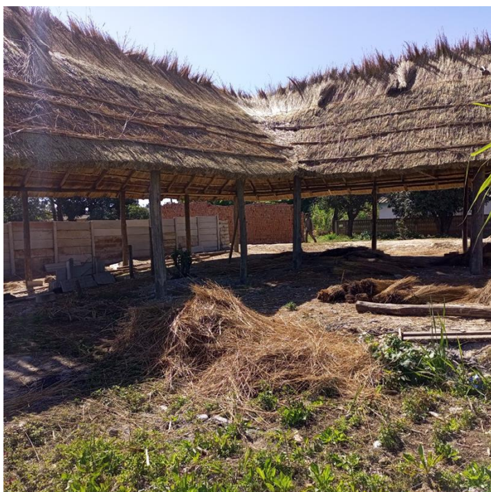
The community hall and cultural center under construction on site, CFHD, 2022
