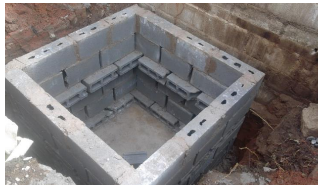
From left leach pit hole before and after the insertion of blocks, CFHD, 2022
